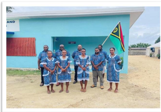
Fig 4.2.15 The completed Santo Office Extension provides an improved working environment for staff.
